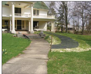
Grass pavers create a ramp without concrete and without altering the historic entrance to the building.
